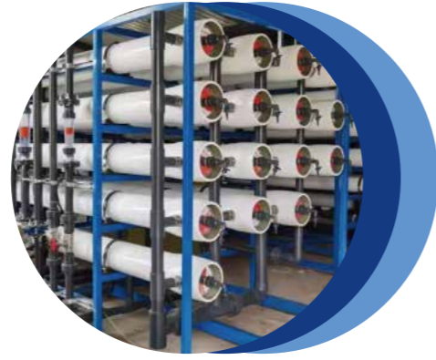
Large-scale Water Plant Project in Anhui Province
