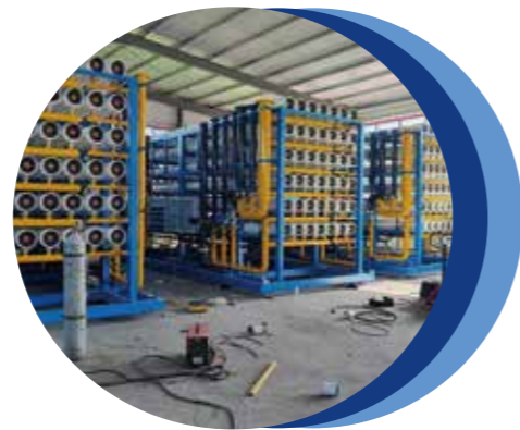
Middle East Industrial Project
