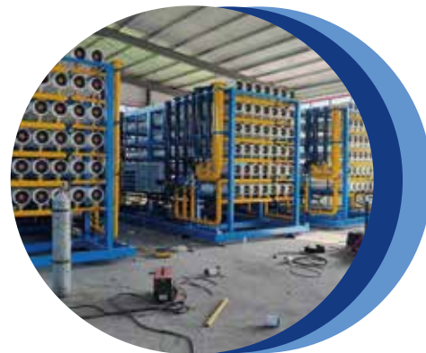
Middle East Industrial Project
